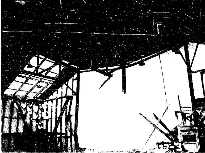
Fig. 3.32 Hangar Building Looking Northwest, Peter Island, Postshot, 15-1/2 Miles from GZ
